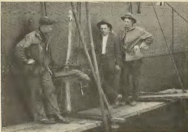
Fig. 3.—Bolting-Up Jack Removing Dent from Ship Plate
